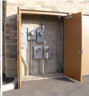
Preferred (utilities inset into the building and behind doors)
